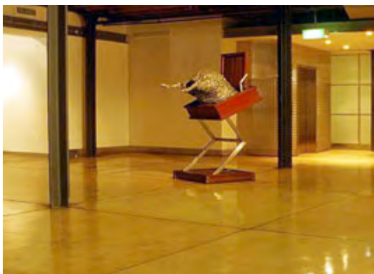
Burnished finish using coloured concrete and clear sealer
